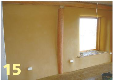
As the work proceeded various repairs and fillers were made using fibreglass. Door, windows frames and sills were masked for protection. Sponge floats produced a smooth finish, which looked like brown sponge rubber moulded around openings.
