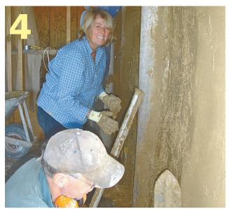
We sprayed the walls with the render pump. We found it best to put one coat on the inside of openings, then do the wall and then add a second coat to the opening for a thick enough coat. We levelled the first coat using screeds. This left a very uneven surface.
