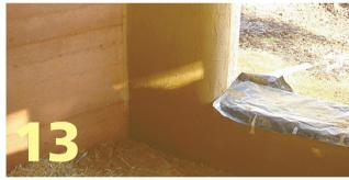
Lower floor wall (split view). The section between the rafters will be above ceiling level. The plastic prevents rain getting between render and wall.
