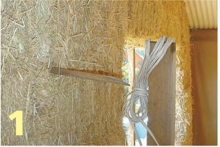
The first thing we did was to fill the gaps between the bales using a thin stick to find smaller holes than my hand could.
