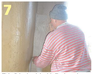
We levelled again and placed the fibreglass mesh across the entire wall. We also put fibreglass down the corners of the wall, cutting 'feathers' for added strength. Then we levelled again and came up with the final surface.
