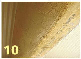
When we redid it, we used a Frank Thomas technique to staple the fibreglass mesh to the wood frame, cob, and then pull the mesh over the cob and work it in as usual. It is much stronger. If we had our time over again, we would do it this way.
