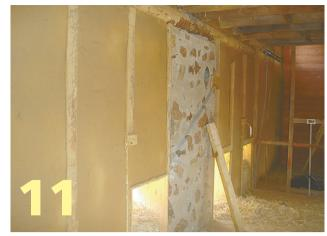
We filled the wheelbarrow and a metal tray with render and completed levelling, putting the fibreglass mesh in and smoothing the surfaces by hand. This shows the final result (without the final coat and paint).
