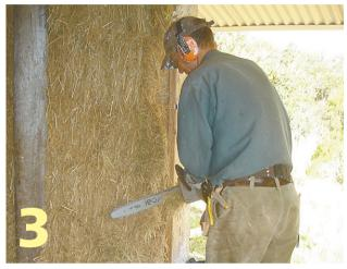
Next we pruned the walls with the hedge trimmer. It sometimes pulled straw out that had not been put in using the 'twist' method. For the fill (as against the bales) we used a pair of hand shears which were more effective.
