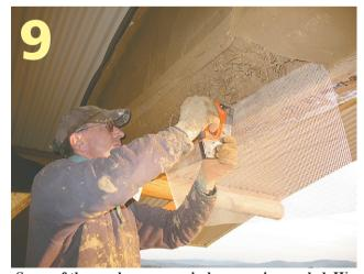
Some of the render over a window opening peeled. We cut away the layers of fibreglass and render and then started this bit again.
