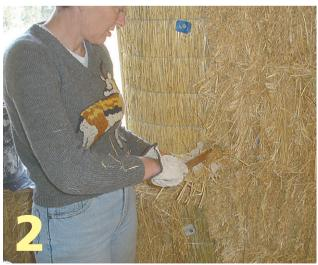
We found that twisting a handful of long straw was best: folding it in half and pushing it into the gaps with the stick. This filled smaller spaces, got more straw in further, and stayed in better.
