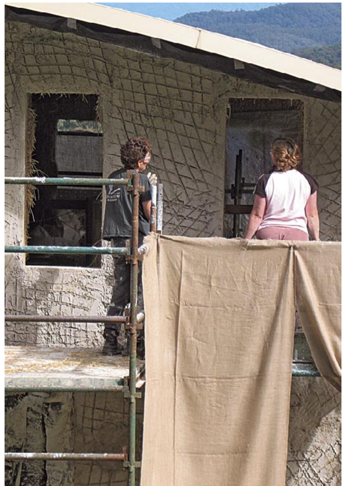
Cross-hatching the first coat.
