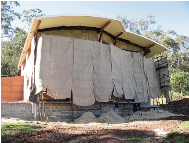
Hessian prevents the render from drying too quickly.
