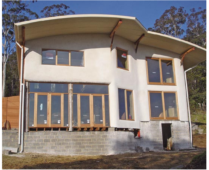
Front view showing plastic form achievable with strawbale construction.
