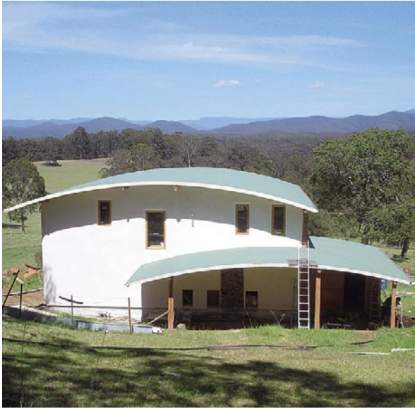
Rear view before final colouring.
