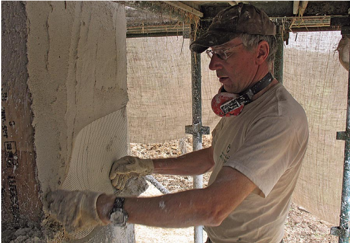
Attaching a layer of fibreglass mesh.
