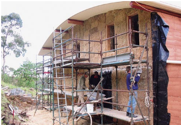
Coating timber in preparation for render.
